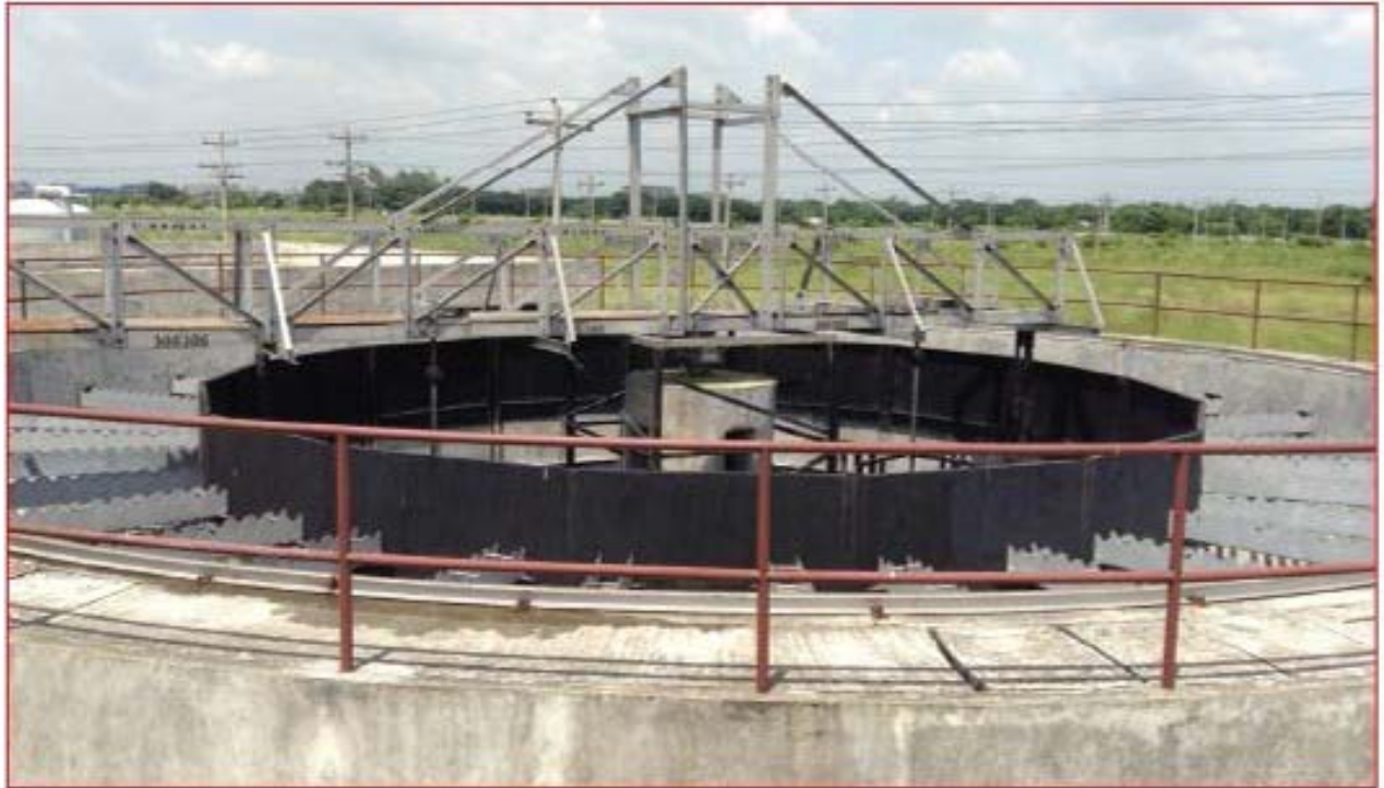
5 Million Gallons per day Water Treatment for Tannery Project for BSCIC at Hemayatpur, Savar, Bangladesh.
